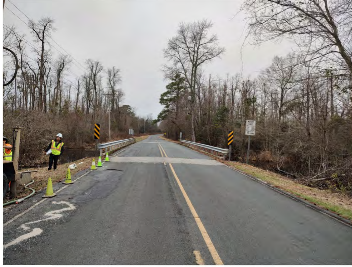
PHOTO 1: VIEW FACING DOWNSTATION FROM END BENT 2.
