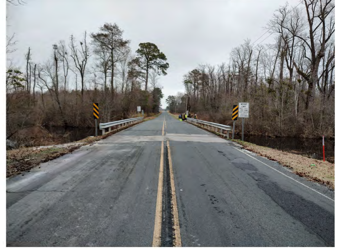
PHOTO 2: VIEW FACING UPSTATION FROM END BENT 1.
